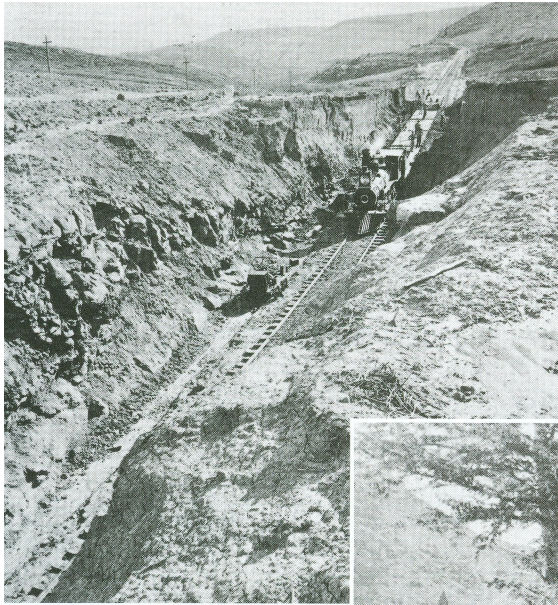
A UP construction train passes through the cut at the head of Echo Canyon. The view is to the east.
